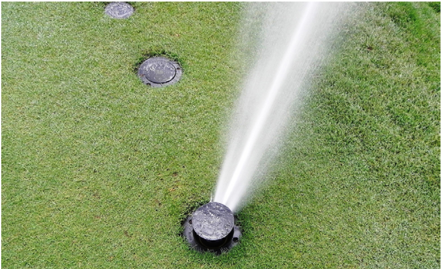
Are sprinkler heads above or below grade? Level sprinkler heads are essential to optimize water conservation and distribution uniformity.
